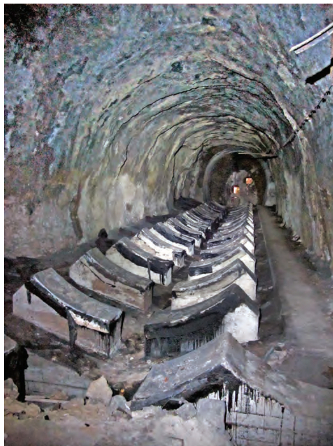
View along World War II tunnel, showing the concrete and bitumen supports for the now-removed fuel storage tank
